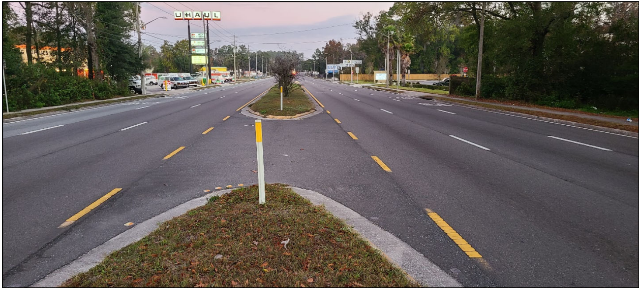
Median Access on S.R. 21 (M.P. 3.455); looking north during the AM peak. Project site is on the left.
